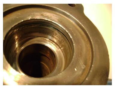
At left can be seen the recess for the seal in the ram housing. The upper groove carries the retaining circlip. With the Chapman seal it is important that the walls of this recess are smooth to aid sealing with the seal's outer 'O' ring.
